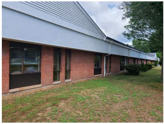
Typical Office/Classroom Window System and Asbestos Cement Soffits
